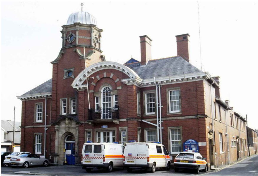
Police Station, Bannister Street, Lytham 30.04.2000 (photo David Forshaw 01)
