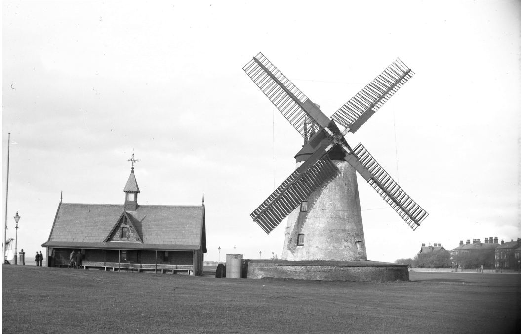
The Mill and Lifeboat House of 1863. The Mill has dispensed with sail cloth and now has the long 'modern' patent sails. These have wooden slats the angle of which could be adjusted by levers. (Think of a Venetian blind in a house or office.) (Lytham Heritage Group)
